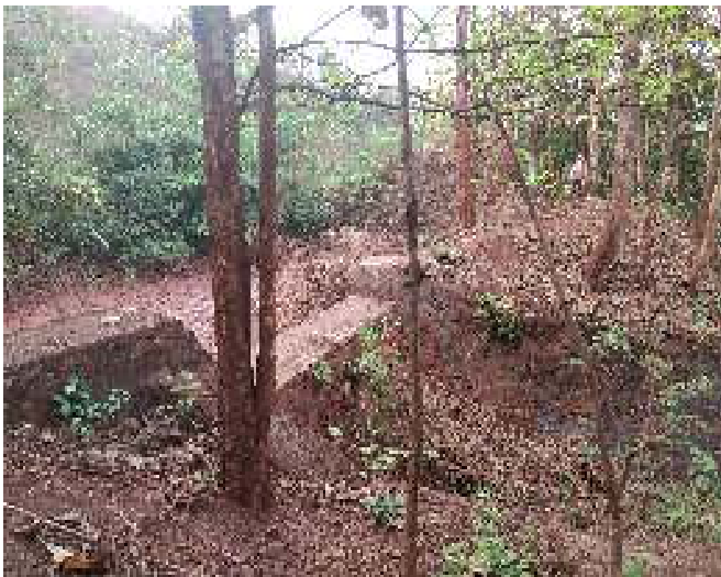
Pic-3: Settling Pond & Check Dam
