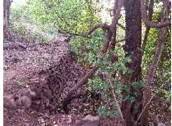
Pic-6: Guard wall along the Nallah
